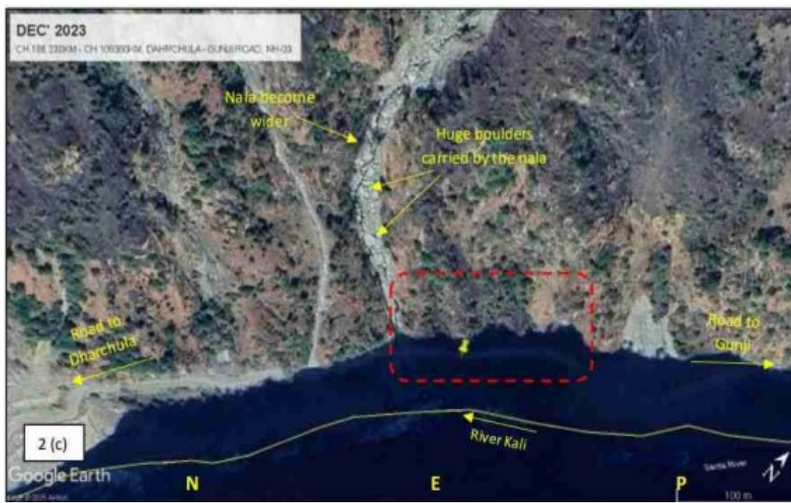
Site View Landslide Loc Ch. 106.230 Km to Ch. 106.360 Km (NH-09) ON P-T ROAD
