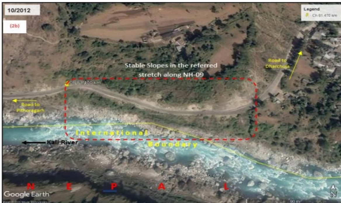
Site View Landslide Loc Ch. 81.450 Km to Ch. 81.755 Km (NH-09) P-T ROAD
