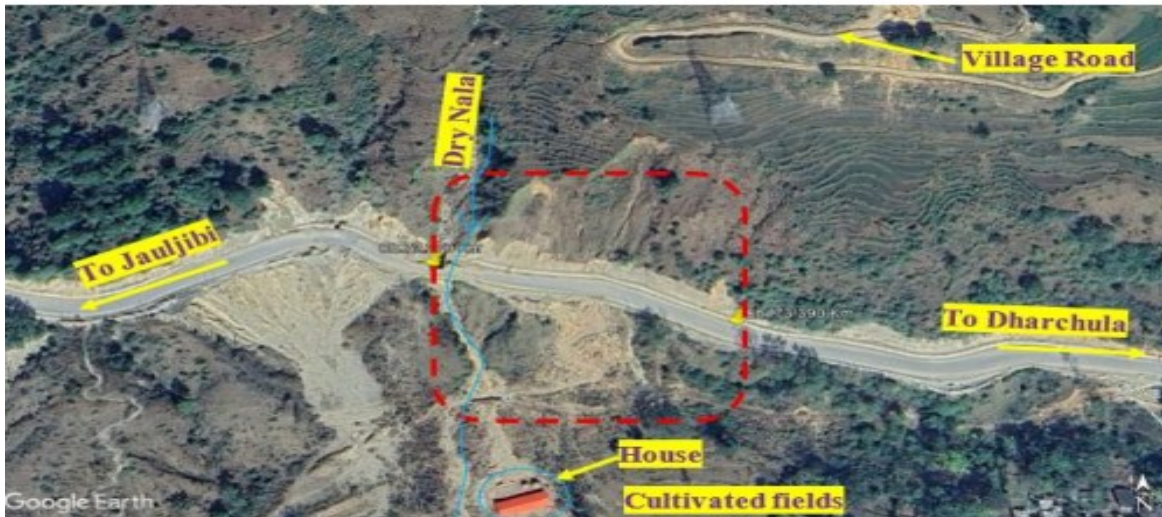
Site View Landslide Loc Ch. 73.270 Km to Ch. 73.370 Km (NH-09) ON P-T ROAD
