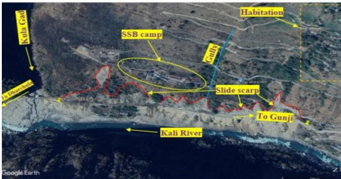
Site View Landslide Loc Ch. 100.465 Km to Ch. 101.425 Km (NH-09) ON P-T ROAD
