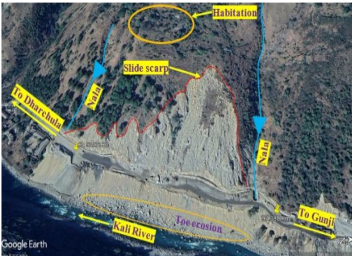
Site View Landslide Loc Ch. 97.040 Km to Ch. 97.415 Km (NH-09) ON P-T ROAD
