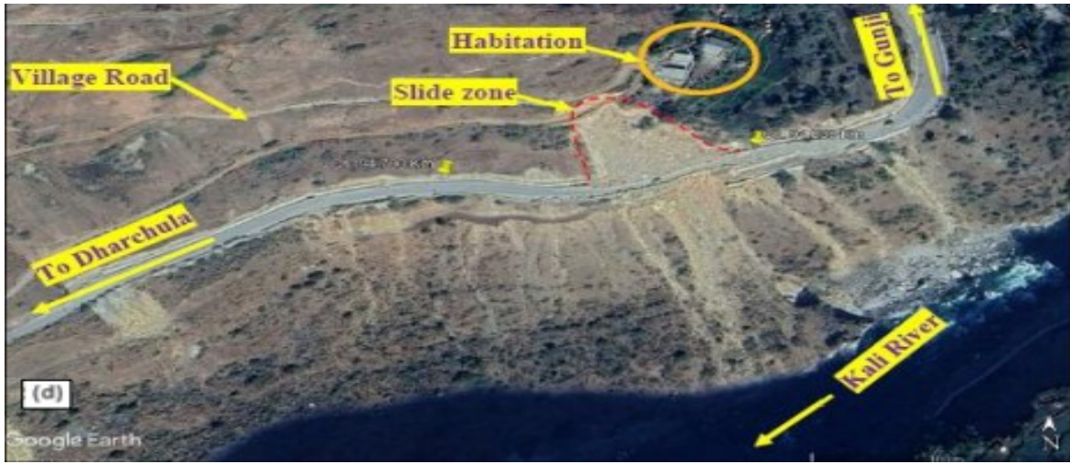
Site View Landslide Loc Ch. 94.720 Km to Ch. 94.830 Km (NH-09) ON P-T ROAD
