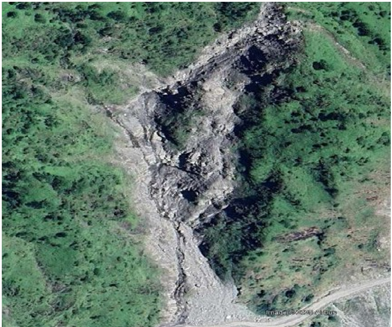
Site View Landslide Loc Ch. 4.680 Km to Ch. 4.880 Km (NH-09) ON T-G ROAD
