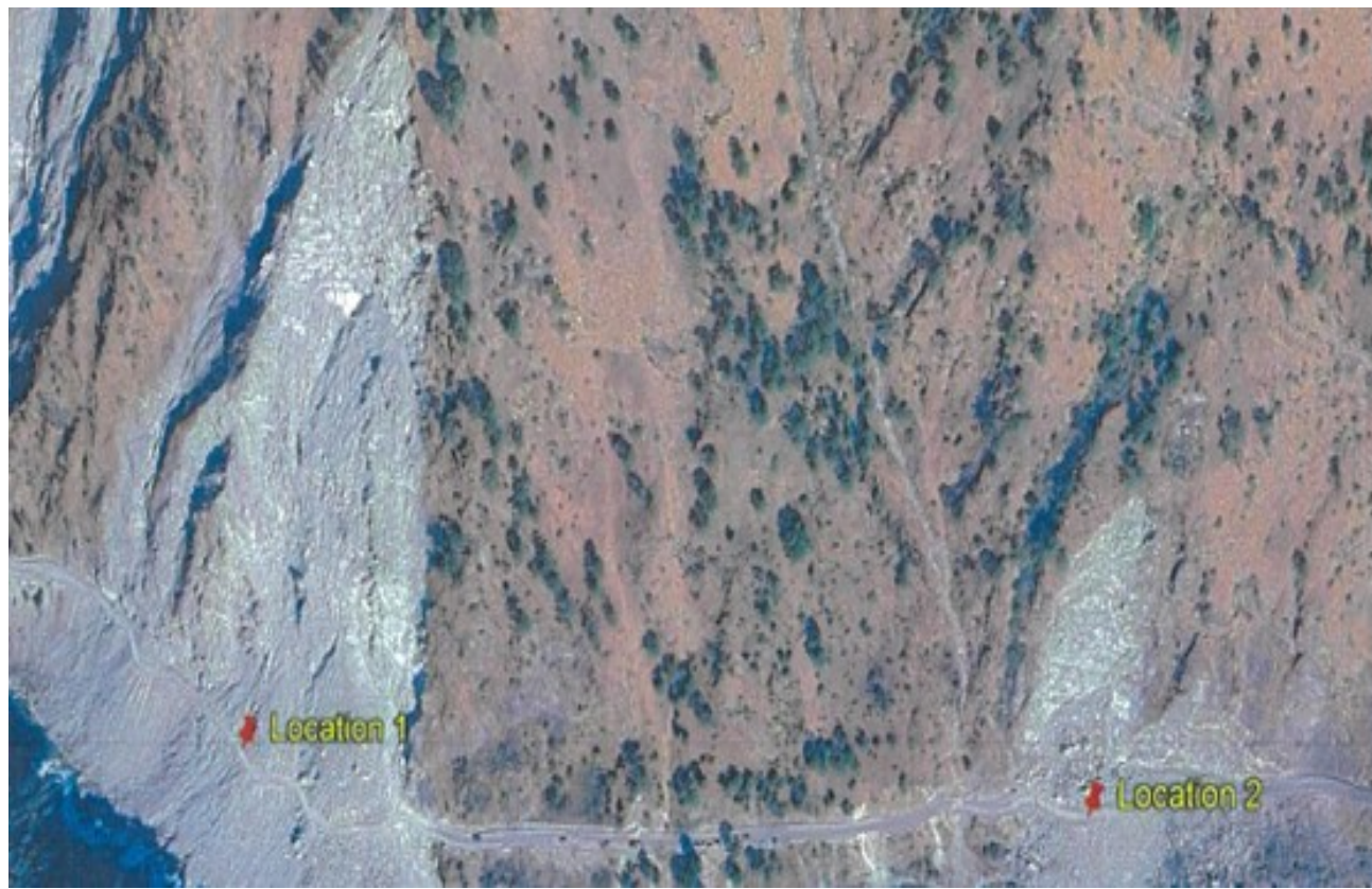
Site View Landslide Loc Ch. 4.890 Km to Ch. 5.250 Km (NH-09) T-G ROAD
