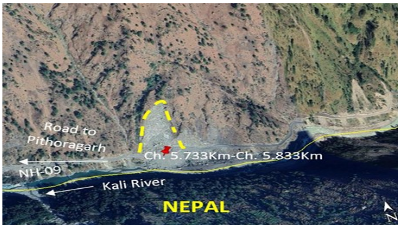
Site View Landslide Loc Ch. 5.733 Km to Ch. 5.833 Km (NH-09) ON T-G ROAD
