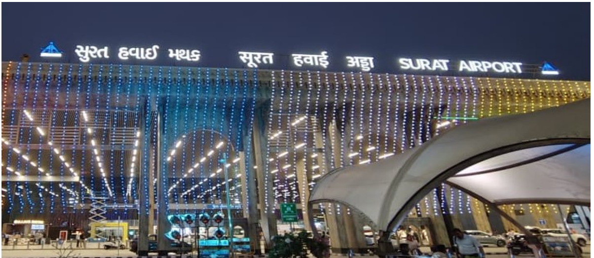
Figure 2: Existing Terminal Building Announcer Signage (Front side)
