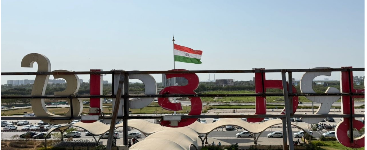
Figure 5: Existing Terminal Building Announcer Signage (Back side)
