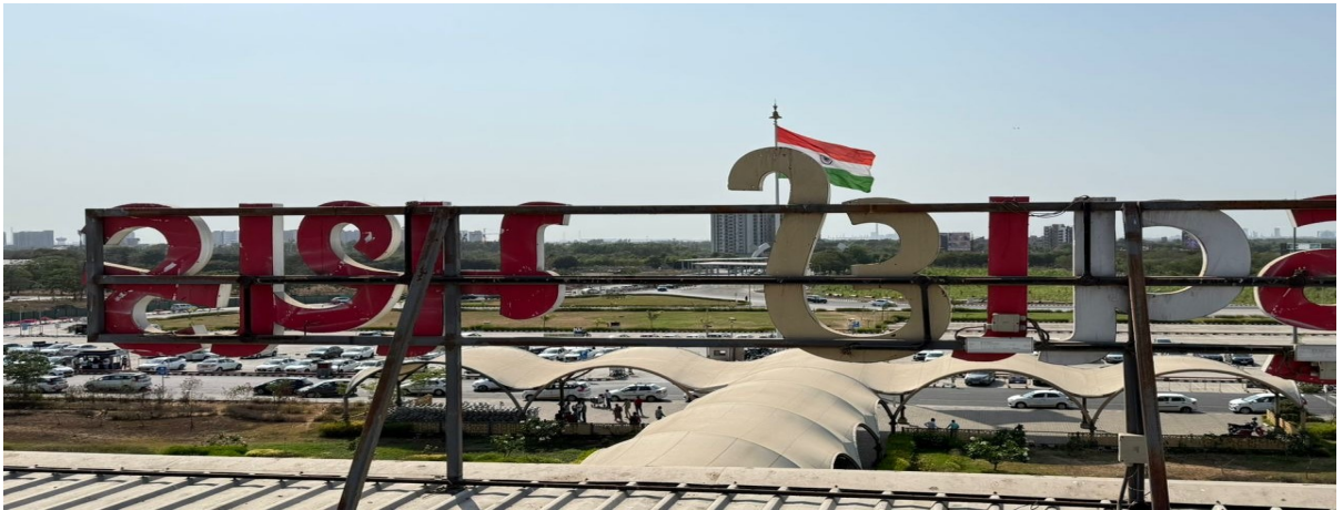
Figure 60: Existing Terminal Building Announcer Signage (Back side)
