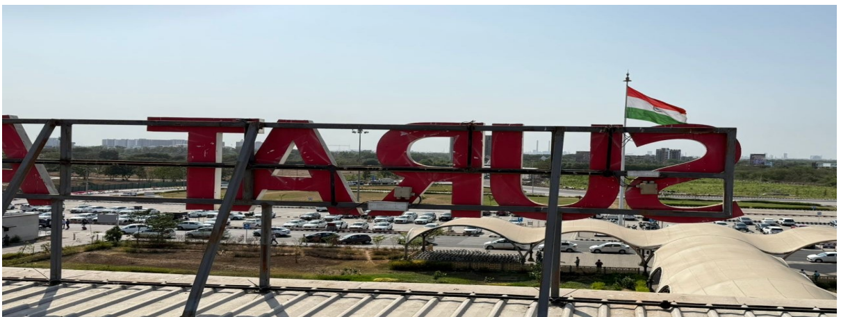
Figure 3: Existing Terminal Building Announcer Signage (Back side)
